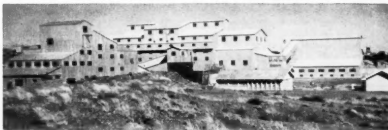
NEW CENTRAL CONCENTRATOR at Kimberley treats ore from three underground mines. Uses both pans and heavy media.
